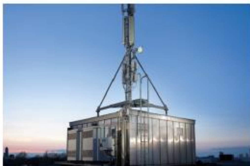
Telecom base stations
